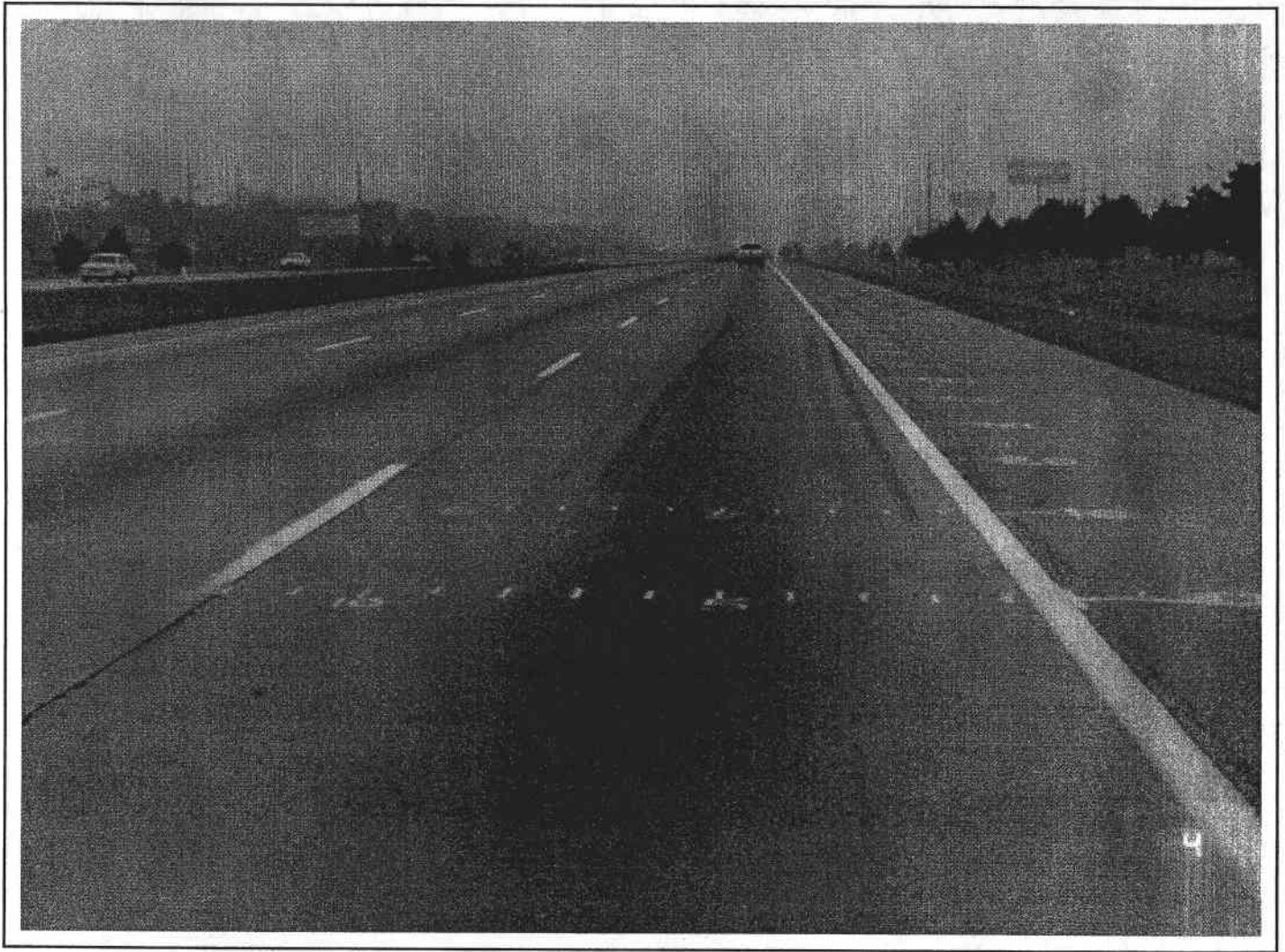
Figure 11 - Pavement markings placed on a busy interstate using spray chalk.
