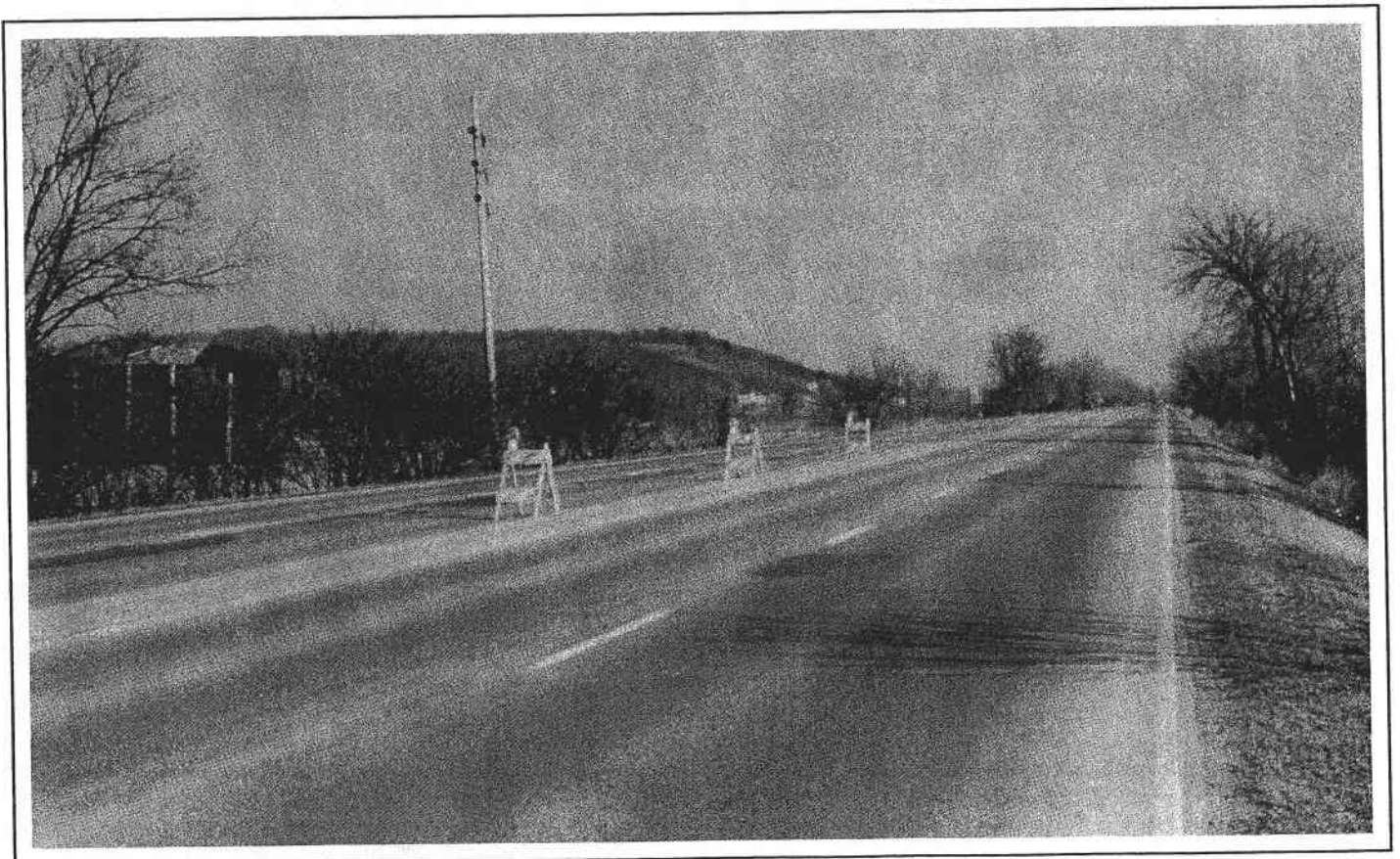
Figure 19 - Same site shown in Figure 18 with barricades set 50 feet apart.
